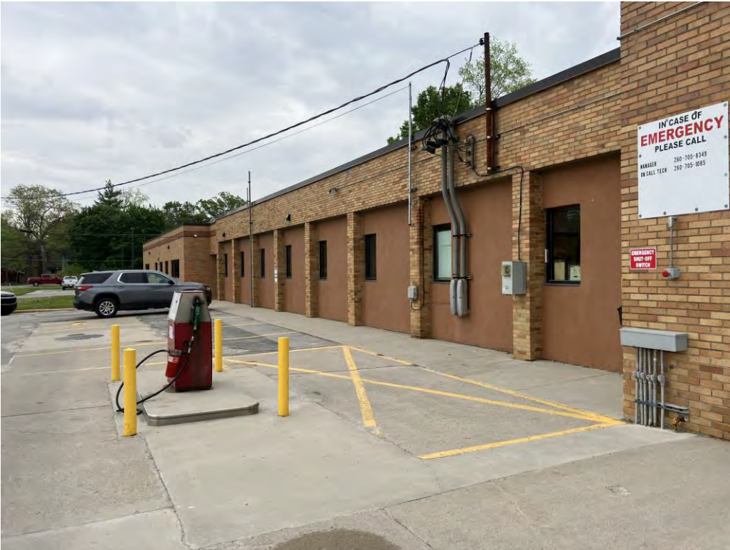
Photo 40: Former garage doors (sealed) on the north side of the building
