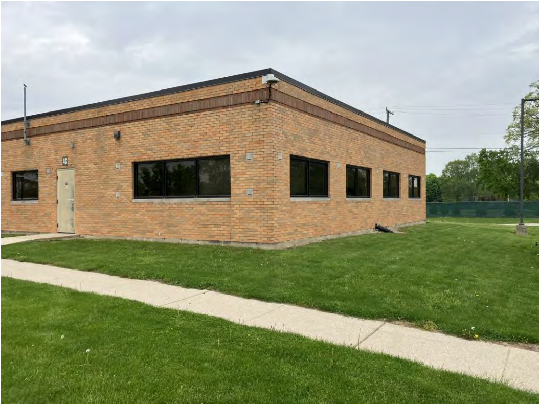
Photo 2: East side of the office/maintenance garage building facing north
