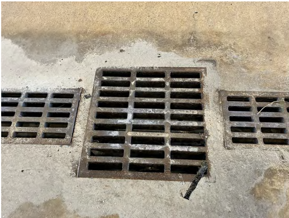
Photo 26: Sump at the wash bay
