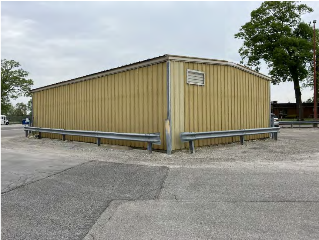
Photo 30: South side of the storage building
