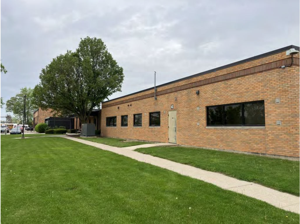
Photo 1: South side of the office/maintenance garage building facing west
