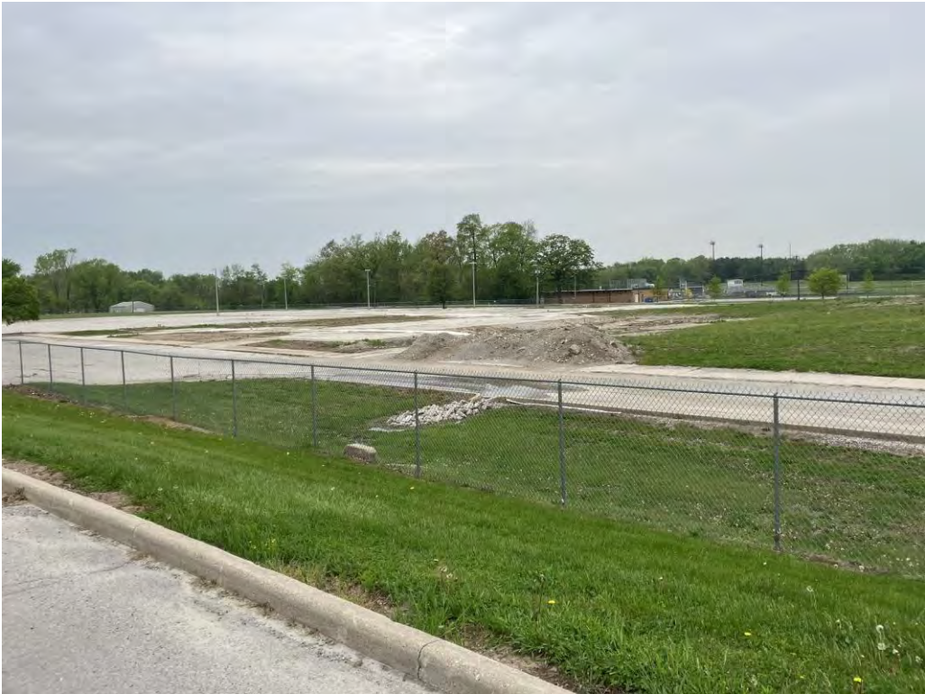
Photo 41: North adjoining property
