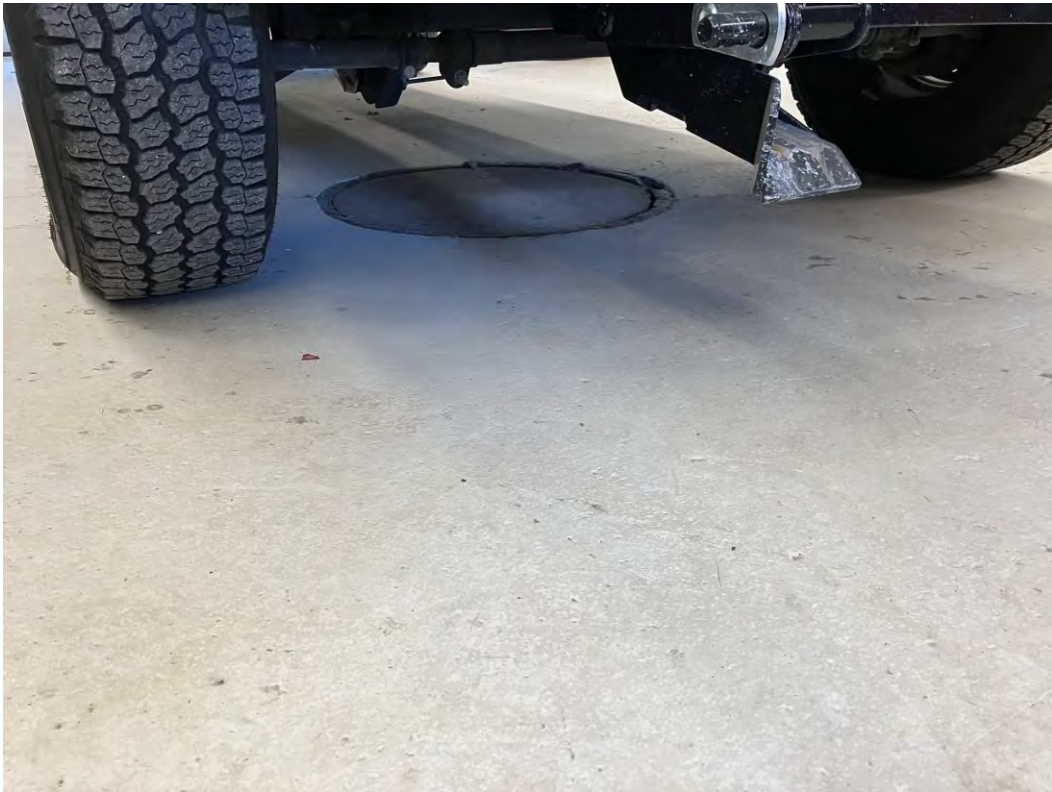
Photo 12: Sump at the east garage bay area
