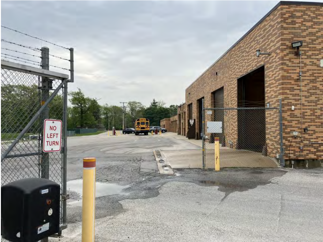
Photo 6: North side of the office/maintenance garage building facing east
