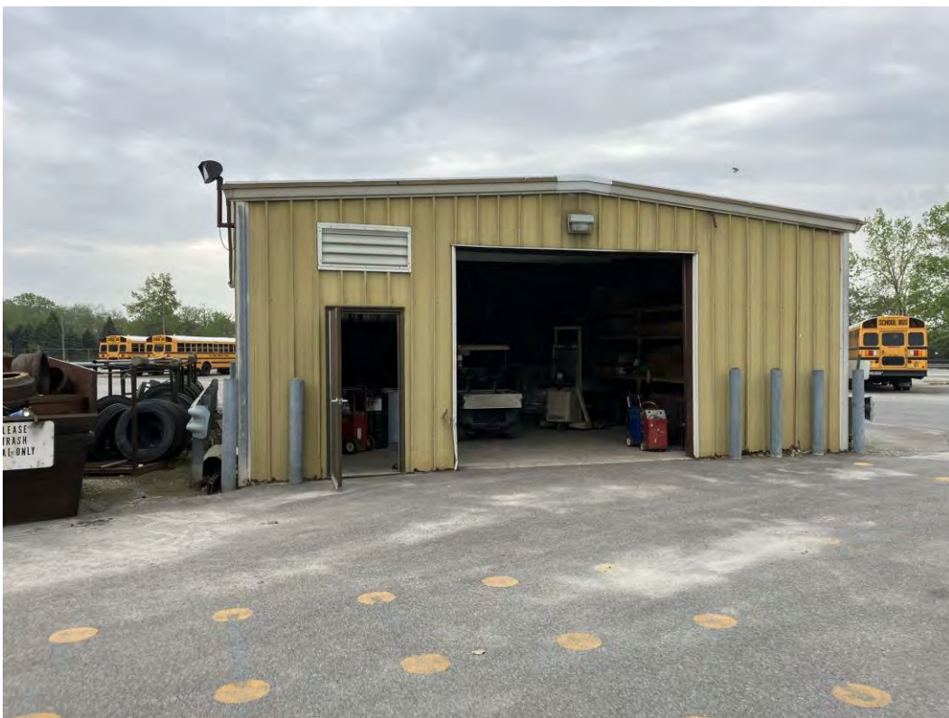
Photo 28: Storage building on the central portion of the property
