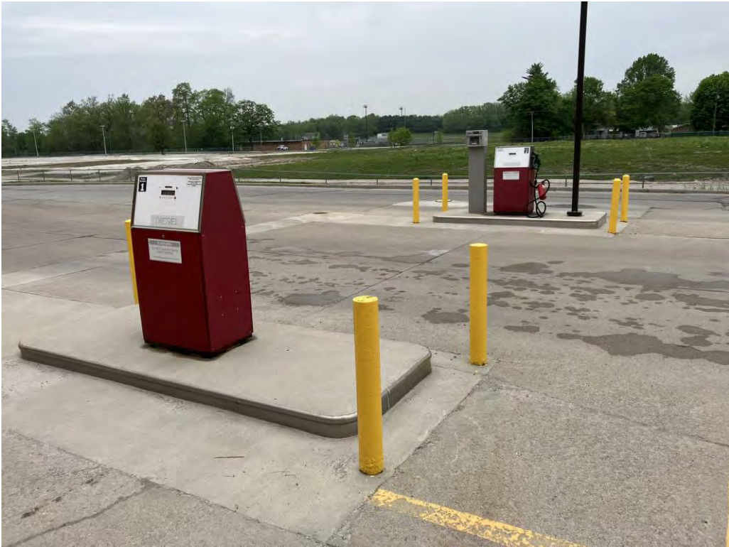
Photo 33: Fuel dispensers north of the building
