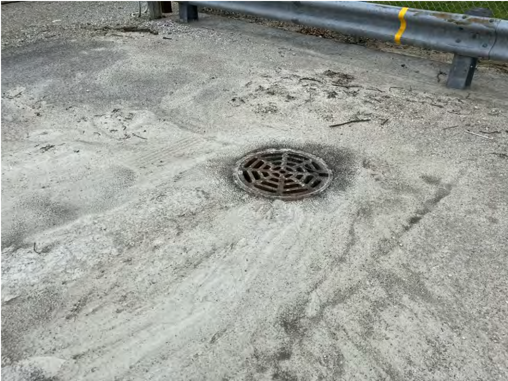
Photo 35: Stormwater catch basin on the northwest portion of the property
