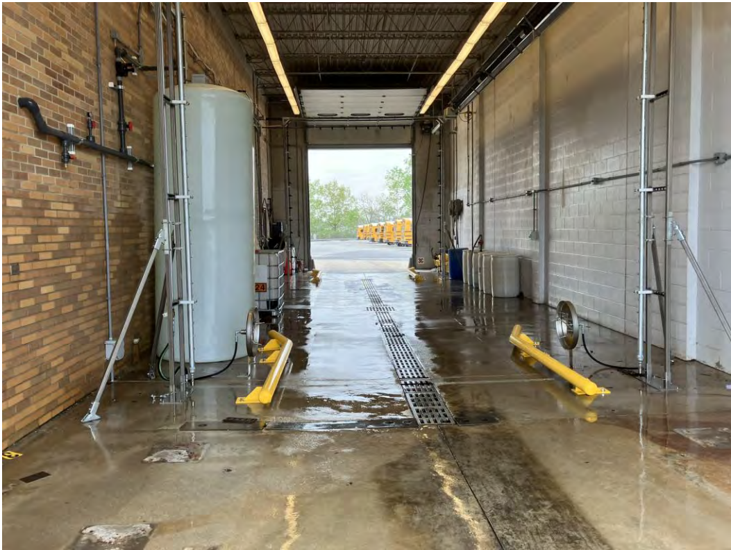
Photo 24: Wash bay in the west portion of the building
