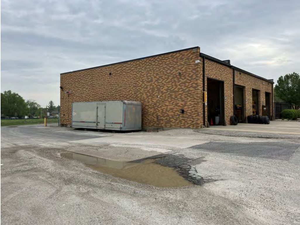
Photo 5: West side of the office/maintenance garage building
