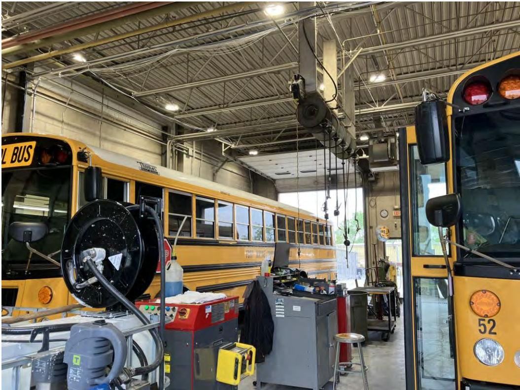
Photo 16: Bus maintenance bays in the central portion of the garage area
