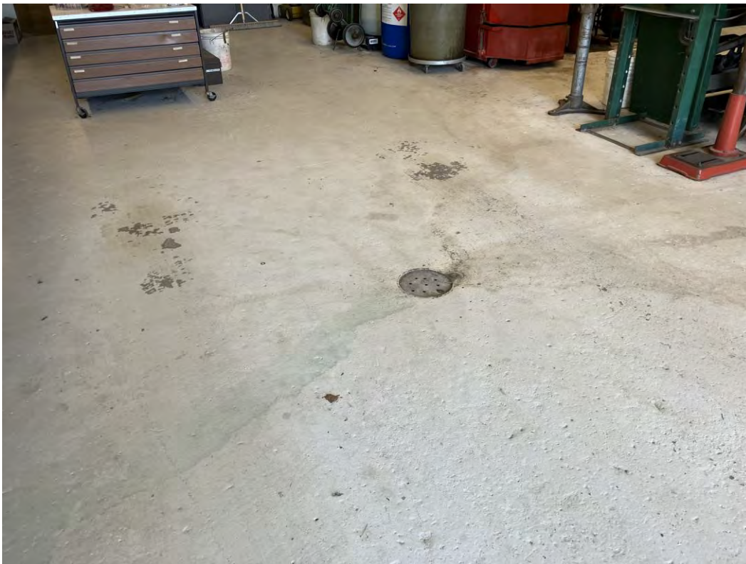
Photo 10: Floor drain in the east garage bay
