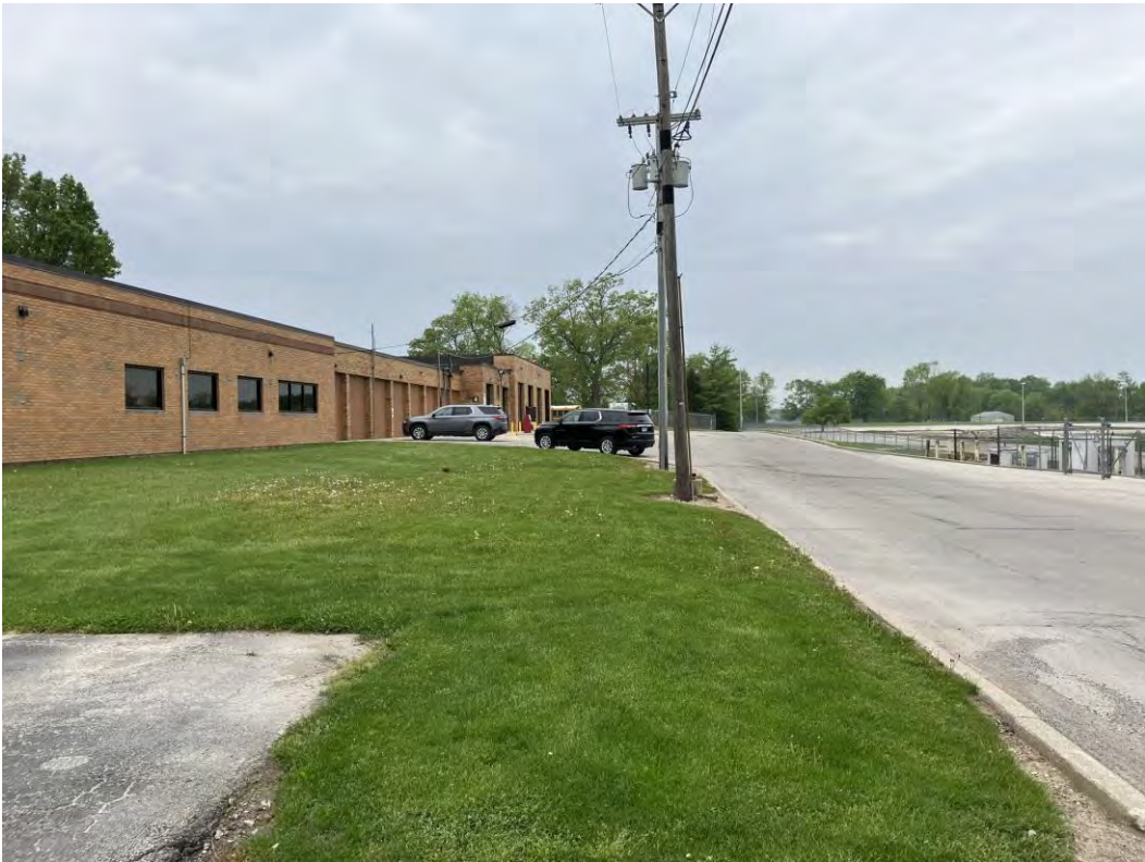
Photo 4: North side of the facility facing west
