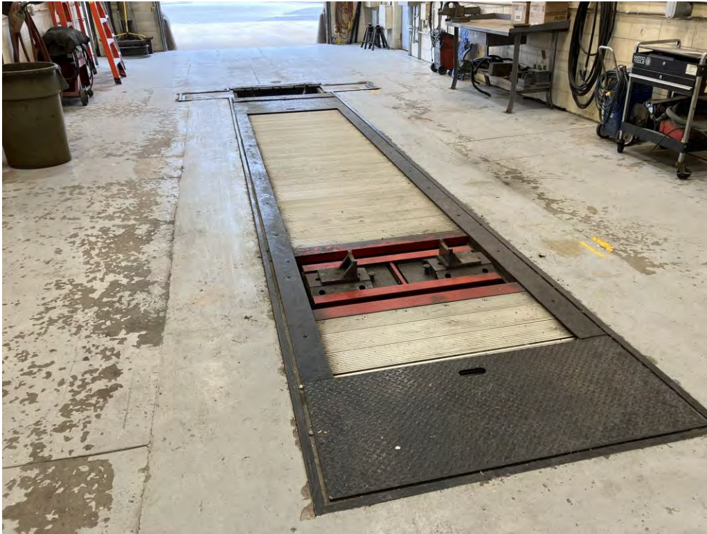
Photo 21: Service pit at bus garage
